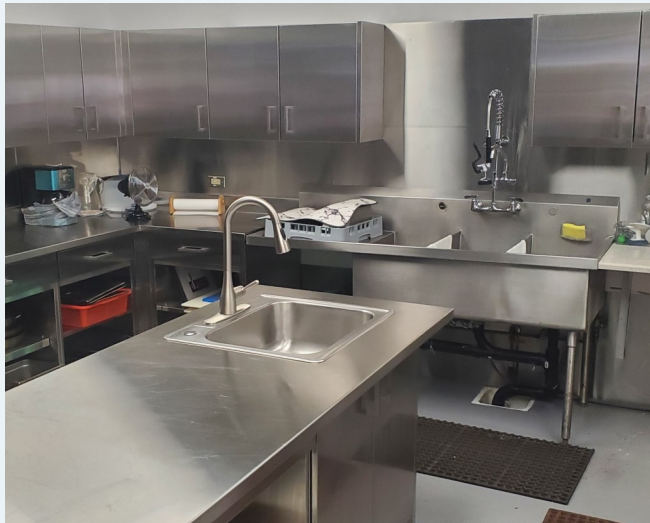
Patagonia Senior Center Kitchen Upgrade
